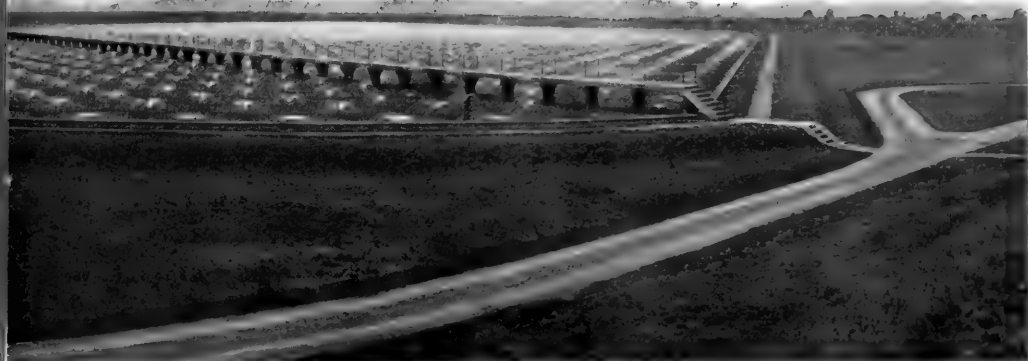
PANORAMIC VIEW OF TRICKLING FILTERS, COLUMBUS, OHIO
