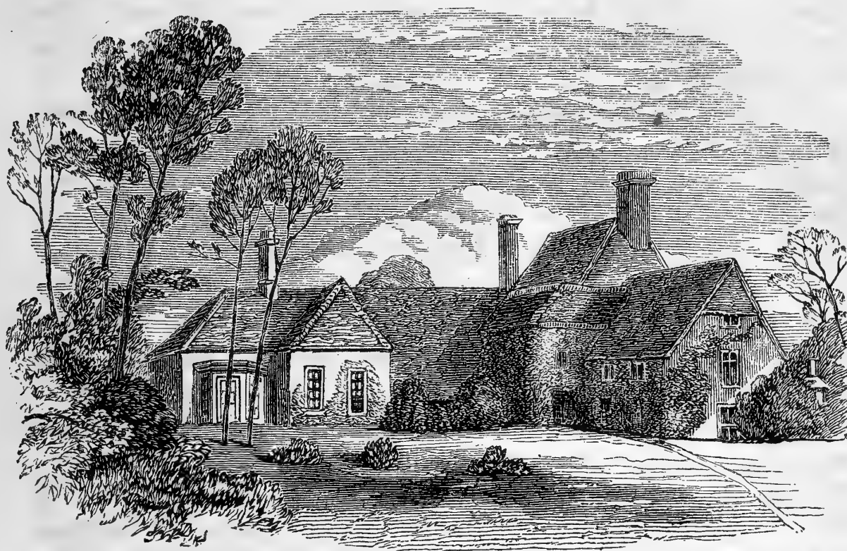
BACK VIEW OF WHITE'S HOUSE.
