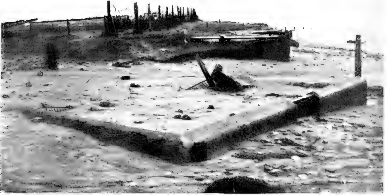
FIG. 1.—Concrete 'Trunk Head,' Stream Dyke. Nov. 12th, 1912.
