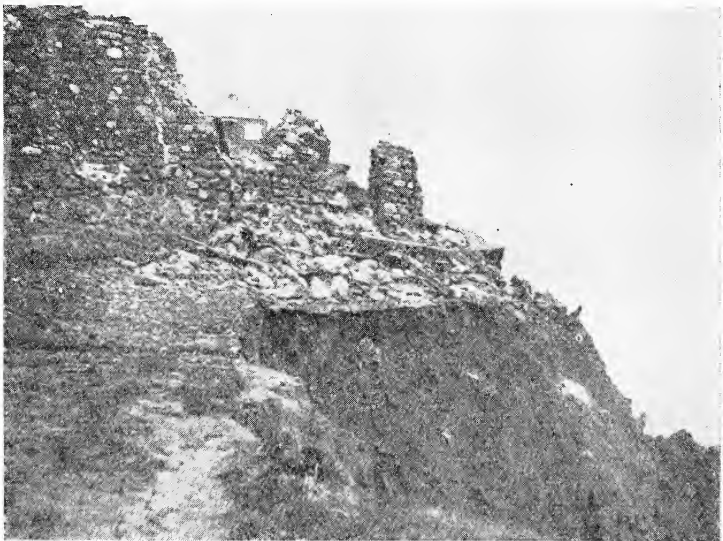
Near View, showing damage to out-building.
