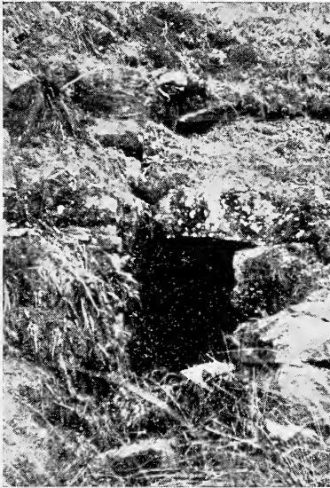
Adit in sound rock, Merryfield Sett, Nidderdale.
