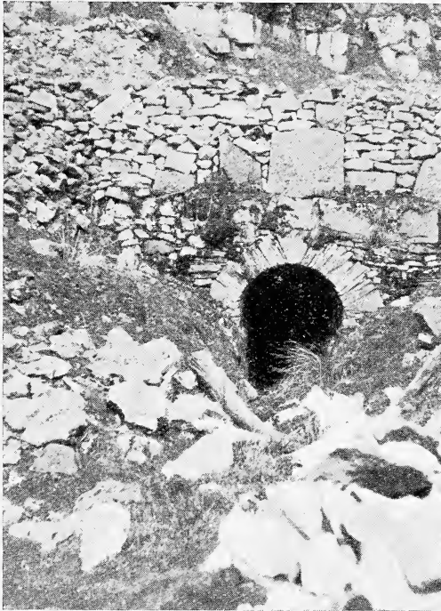
Typical Arch Masonry—in 'bad' ground.
