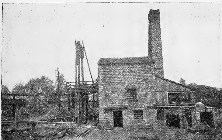
FIG. 10.—Engine House, Denby Grange Colliery, showing gin and capstan on the left.
