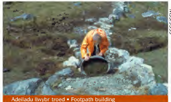
Adeilladu llwybr troed • Footpath building
