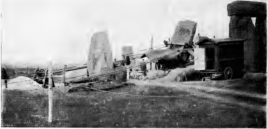
FIG. 1.—The work at Stonehenge. Raising the leaning stone.
