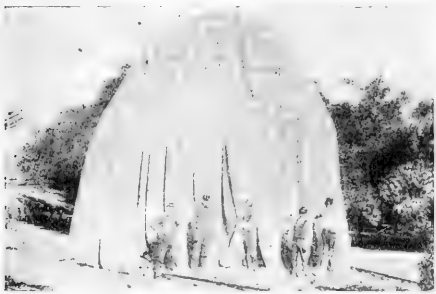
FIG. 2.—Tent in position for fumigation.
