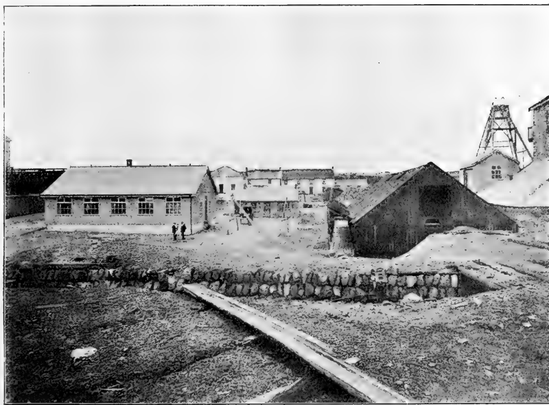
Mine Buildings of Camborne Mining School, Cornwall.
