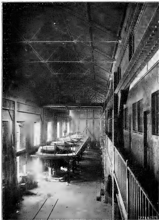
FIG. 1.—The British Aluminium Company's Power-house at Foyers.
