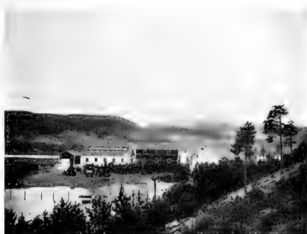
FIG. 1.—View of nitric acid factory at Notodden.
