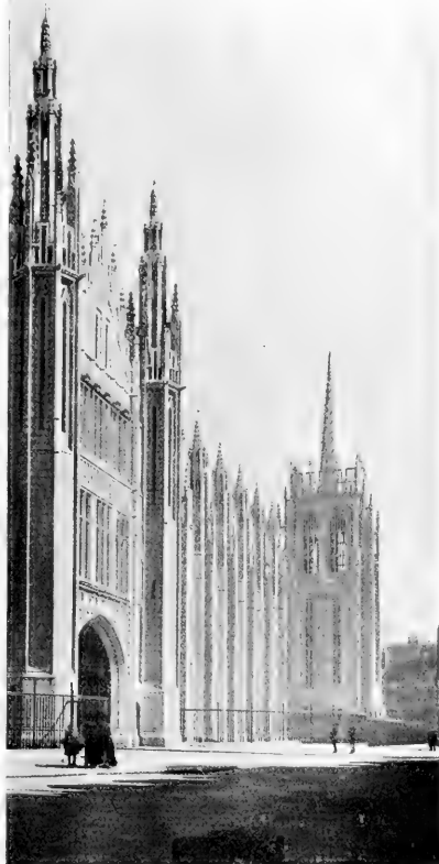
FIG. 2.—Front of Marischal College Buildings, looking southward.
