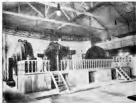
FIG. 4.—Photograph of three 500-kilowatt furnaces at Notodden.
