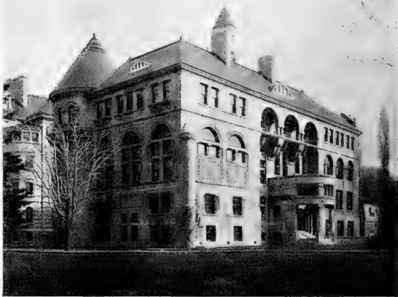
FIG. 1.—Macdonald Physics Building, McGill University, Montreal.
