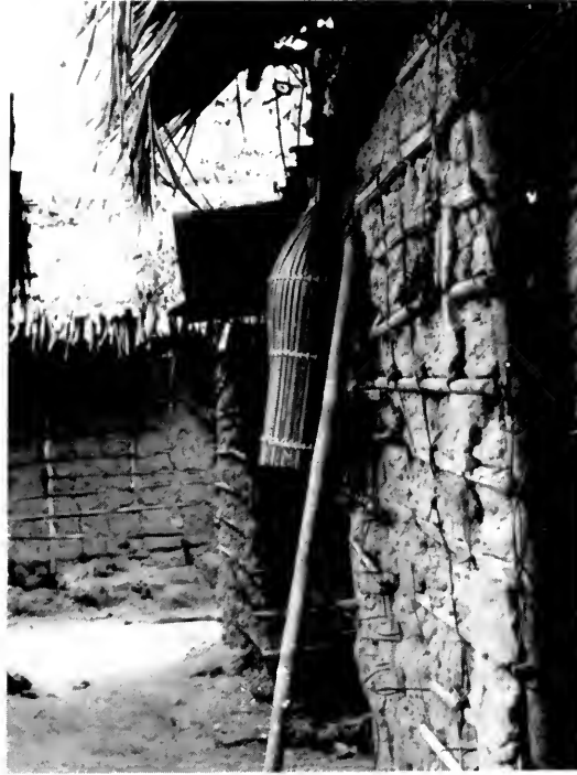
Mudswitch houses with Raphia roof. Fish trap made from Raphia petioles and cane. Photo : J. Falconer
