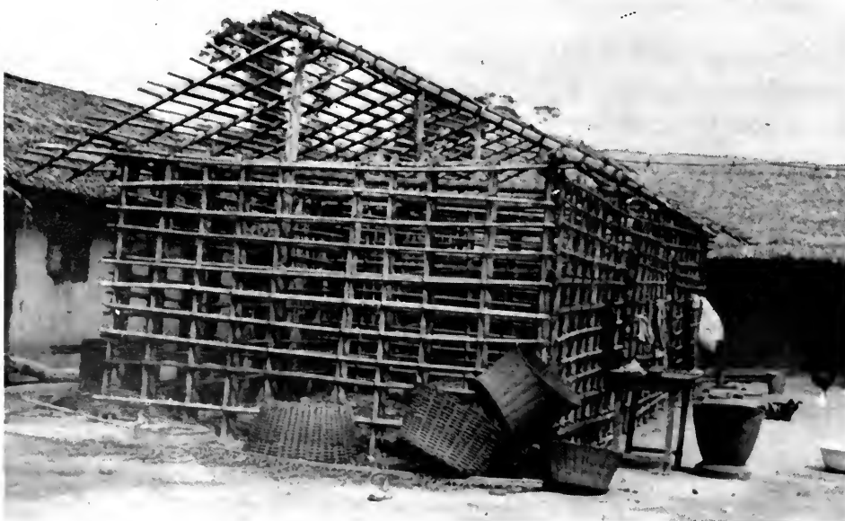
Frame of mud switch house with tree poles and Raphia rachis
