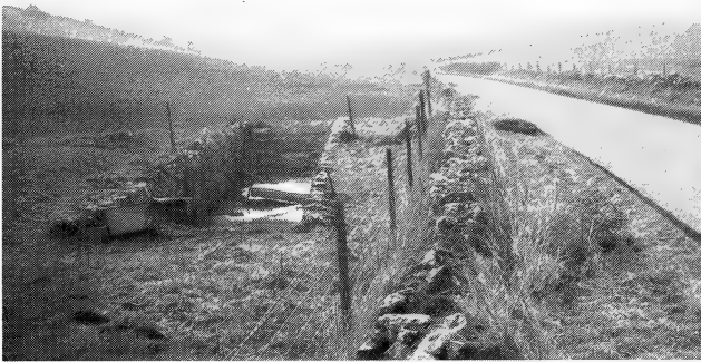
FIGURE 4. Derelict stone-built pond once fed by runoff from the road down a dry valley. Kingdown Farm.
