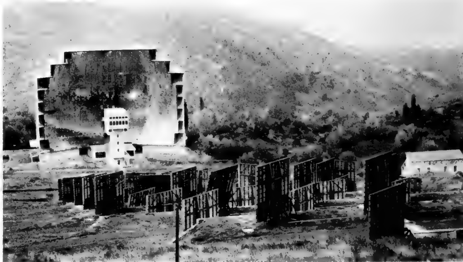
The world's largest solar furnace, built on a hillside in France, has over 20,000 mirrors that bring so much sunlight together at a small spot that its heat can melt a hole in a half-inch-thick steel plate in less than a minute. The flat mirrors on the hillside reflect sunlight to the huge, concave wall of mirrors in the background, which focuses the light on a small area in the tower. Objects can be placed in the tower to see how various materials are affected by high heat—as high as 7,000 degrees Fahrenheit when all the mirrors have been properly adjusted.
