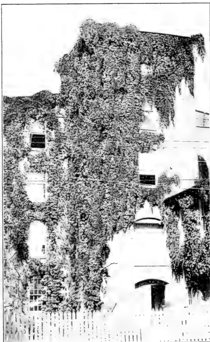
FIG. 156. A FACTORY COVERED WITH WOODBINE
