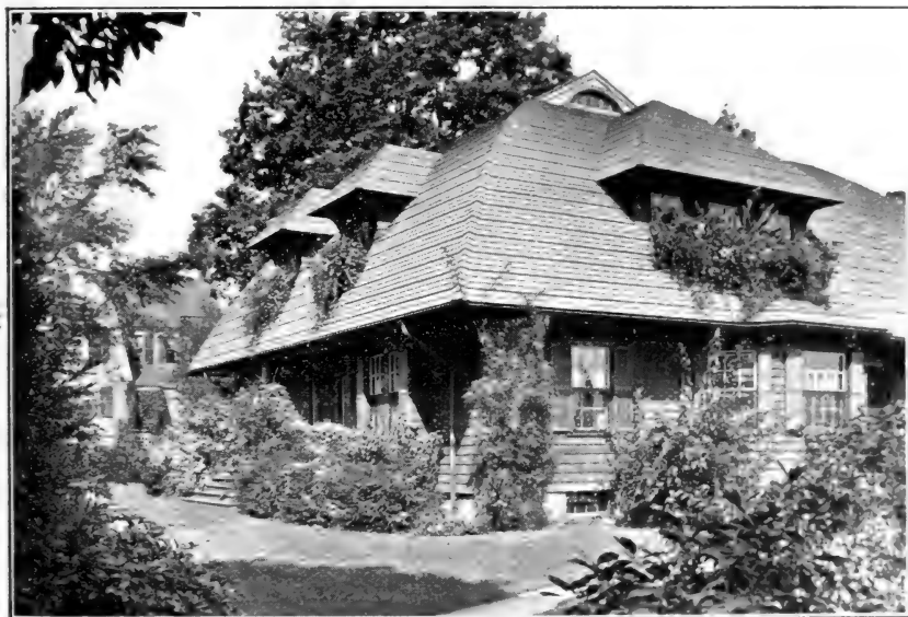
A LOW-ROOFED COTTAGE UNITING WITH THE LANDSCAPE. WHY NOT SUCH ARCHITECTURE AND SUCH PLANTING FOR OUR SCHOOLHOUSES?
