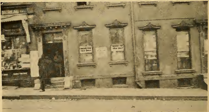
A Typical Boarding House on Lower Wylie Avenue.
