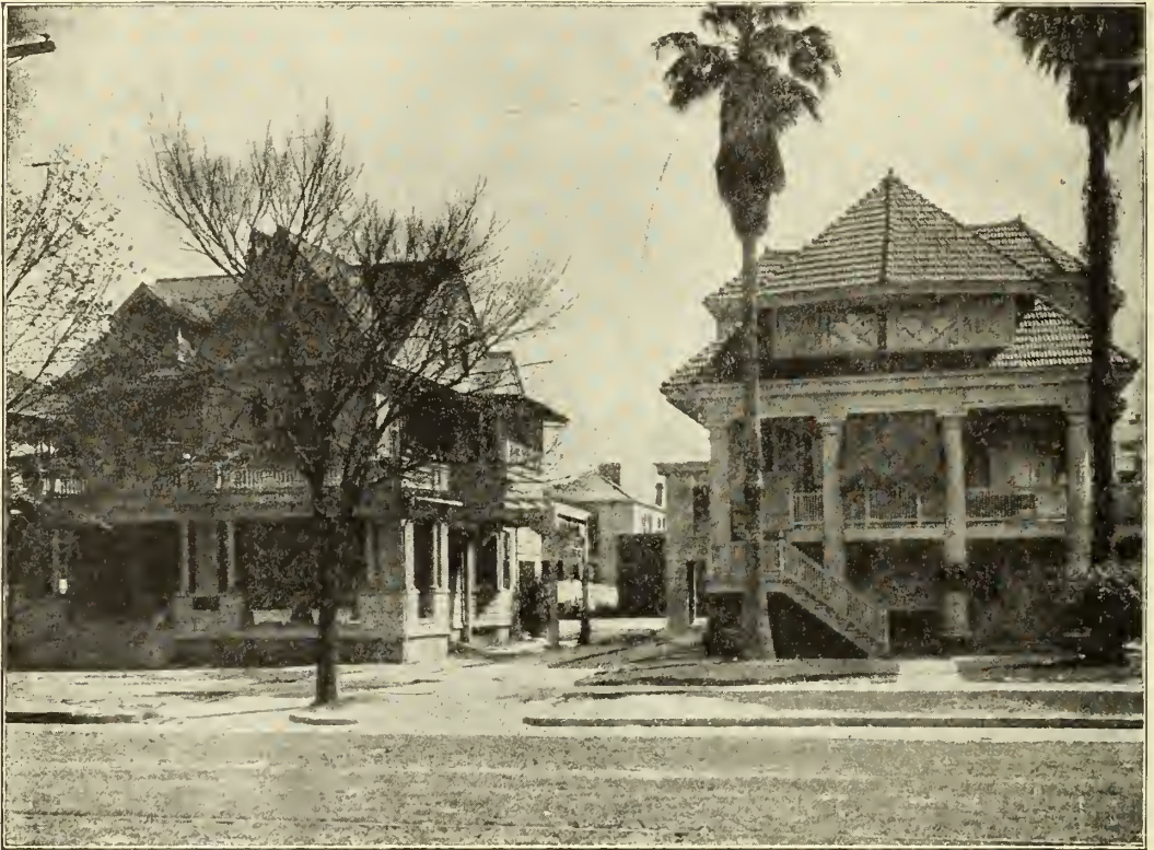
Some of the Clinic Buildings
