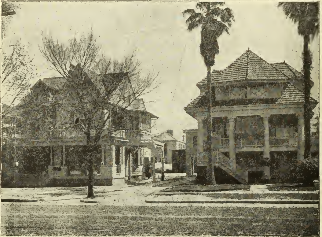
Some of the Clinic Buildings
