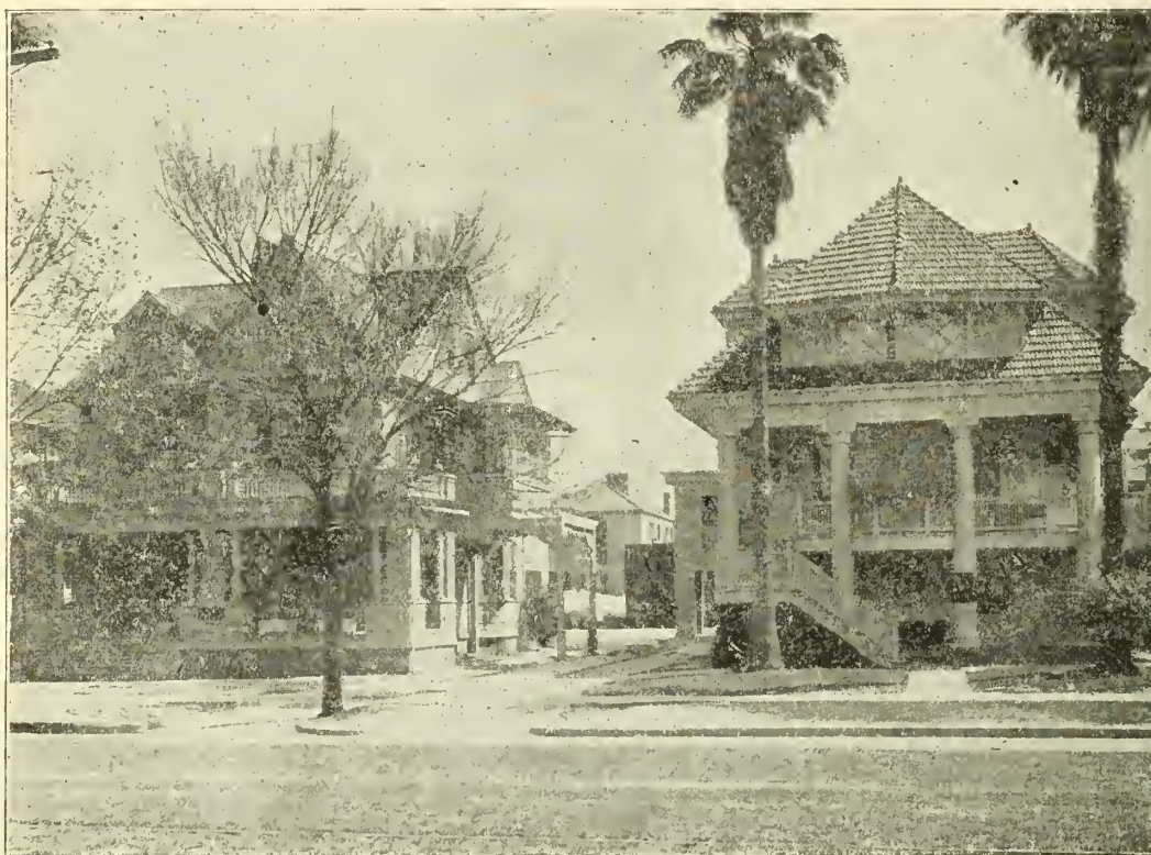
Some of the Clinic Buildings
