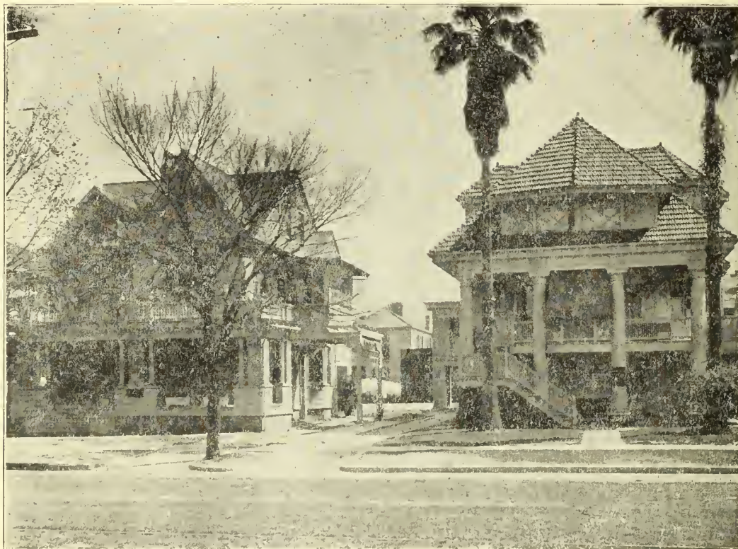
Some of the Clinic Buildings
