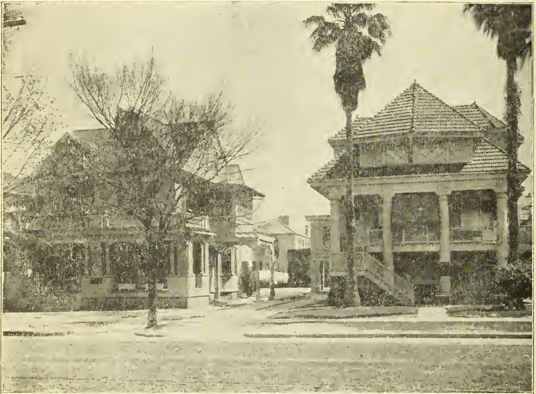
Main Clinic Buildings
