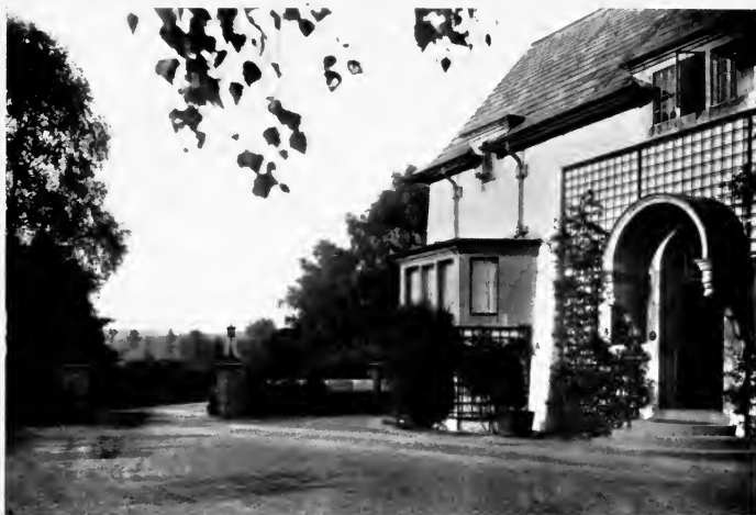
THE ENTRANCE COURT
