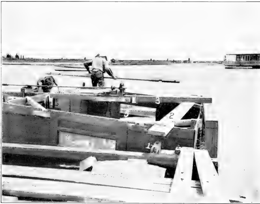
FIG. 10.—The cleats being removed, the car rises part way by its own buoyancy. Opening doors of the slot at end of car to admit the longitudinal shaft beam allows the car to be entirely raised. 1, cleat; 2, holding-down plank; 3, longitudinal shaft beam; 4 and 5, side windows
