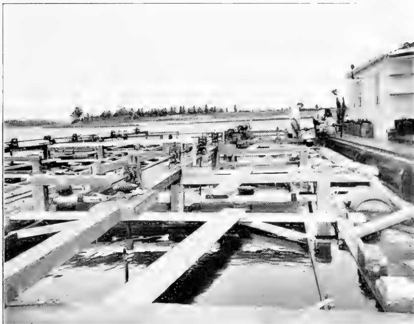
FIG. 3.—Starboard side, looking aft, inside float. Shafting system and general arrangement of cars
