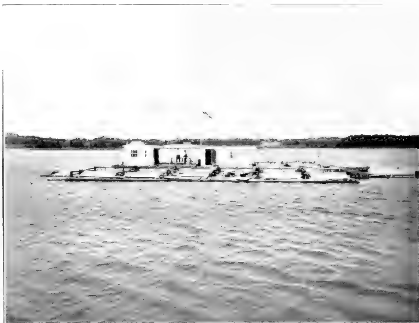
FIG. 1.—Floating laboratory and rearing plant from the port side. The forward (left) house serves as a laboratory and the after one as the engine house and tool room. Most of the rearing cars are covered with white awnings.
