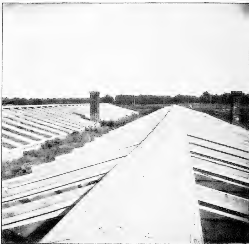
LONG ISLAND SASH HOUSE.
