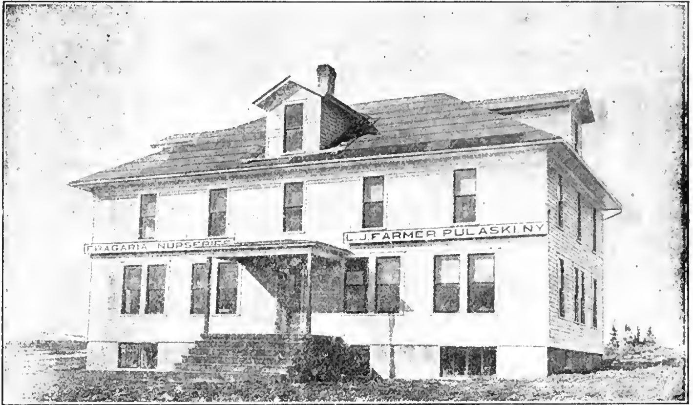
The above shows our Office Building occupying a ground space of 30 by 52 feet
