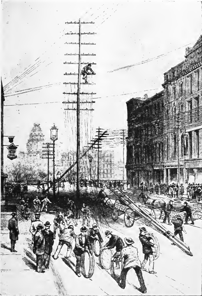
The fight to put telegraph and electric wires underground was a bitter one. Finally, Mayor Grant felled the telegraph pole at the corner of 23rd St. and Broadway with his own hands. The corporations, seeing that he meant business, succumbed to the inevitable.
