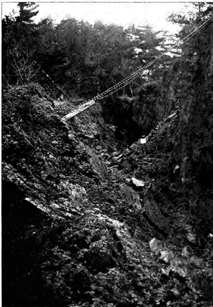
Stockport slide. Open fissure between the downthrown and upraised blocks. Soft clay in bottom extruded from below.
