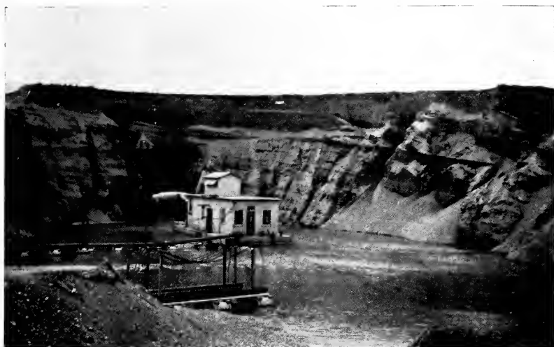
Figure 32 A sand-sucker operation in gently dipping beds of a delta deposit
