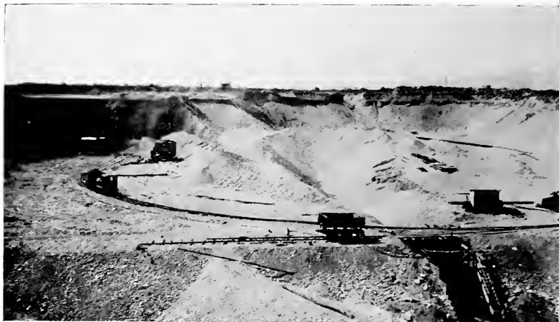
Figure 36 An old glacial river deposit. Pit cars dump into the hopper in the foreground which feeds onto the plant conveyor belt
