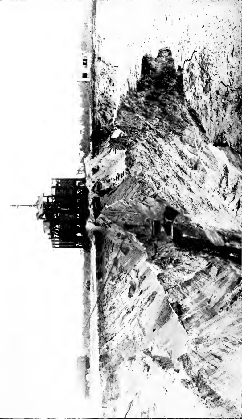
Figure 4 Slack line cableway type of operation
