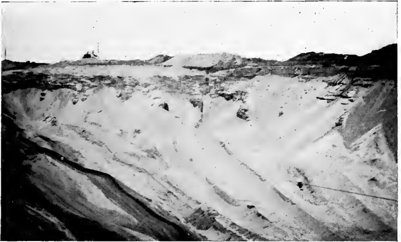
Figure 8 A drag line operation showing the ridges of unexcavated material
