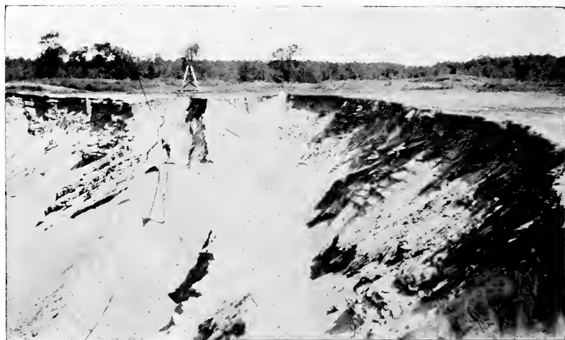
Figure 3 A Sauerman slack line cableway excavating a delta deposit
