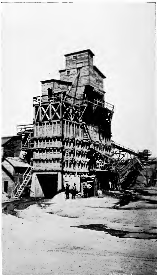
Figure 34 An up-to-date washing and screening plant showing both open stock pile and bin storage. All of the production is hauled by automobile truck
