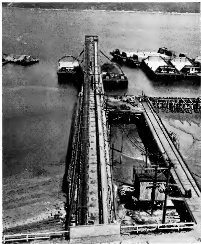
Figure 24 Loading by conveyor belt onto barges
