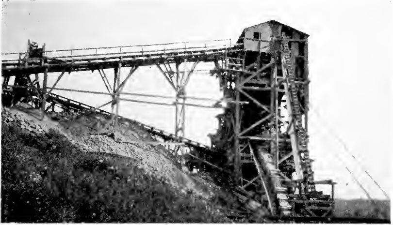
Figure 21 A belt conveyor feeds the material from the pit and a bucket elevator lifts the broken gravel from the primary crusher
