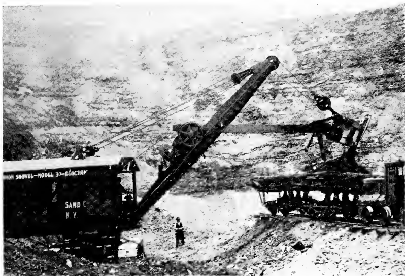
Figure 27 An electric shovel excavating in a cemented, hard delta deposit. The level bedding planes are unusual
