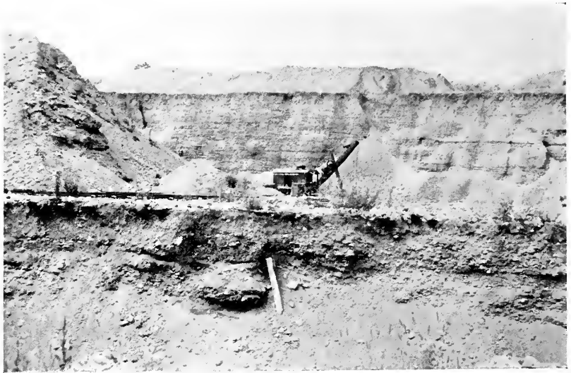
Figure 26 A coarse sand and gravel delta deposit with a total thickness of about 135 feet. The present face is 70 feet in height and two levels will be used to get the entire thickness
