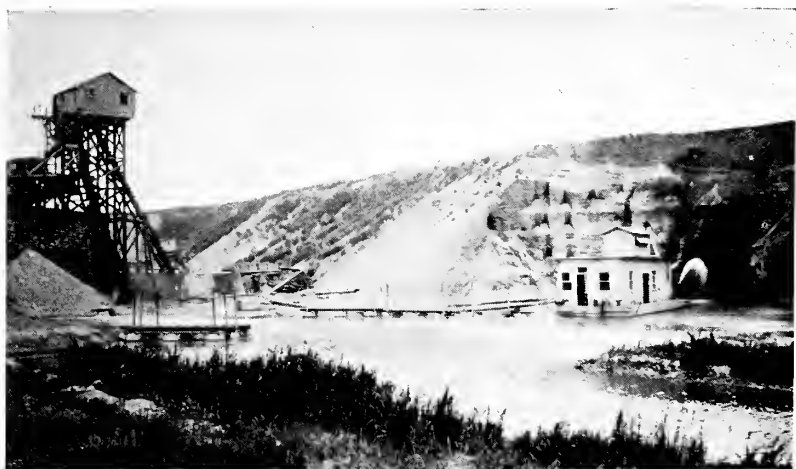
Figure 13 Centrifugal pump excavating a 70-foot deposit which carries 60 per cent of gravel
