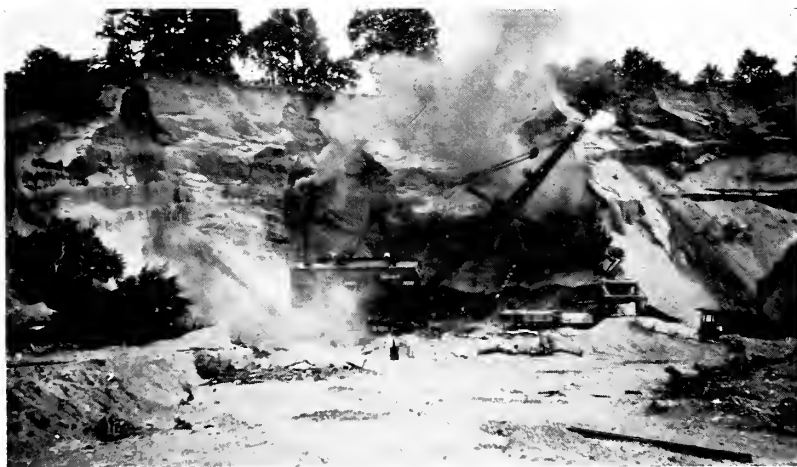
Figure 17 Steam shovel loading a string of pit-cars
