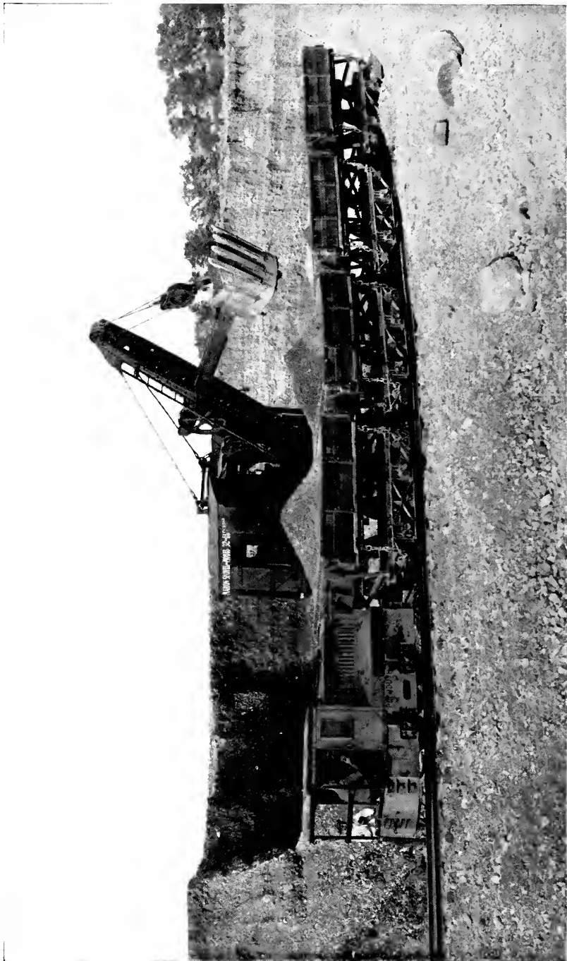
Figure 29 An electric shovel excavating a 25-foot face in a uniformly bedded delta deposit
