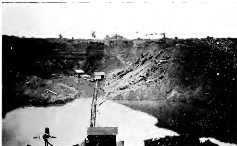
Figure 16 A doubling in production of this six-inch pipe line was secured by installing the booster pump shown in the foreground
