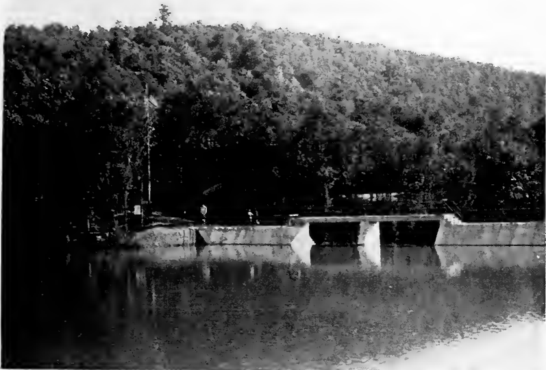
Figure 3 Site of the Allegheny School at the shore of the lake, and hidden among the trees
