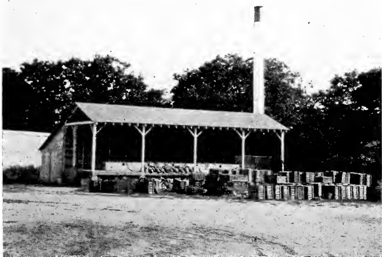
Figure 9 Hot water plant used for the treatment of narcissus bulbs infested with eelworms and bulb flies
