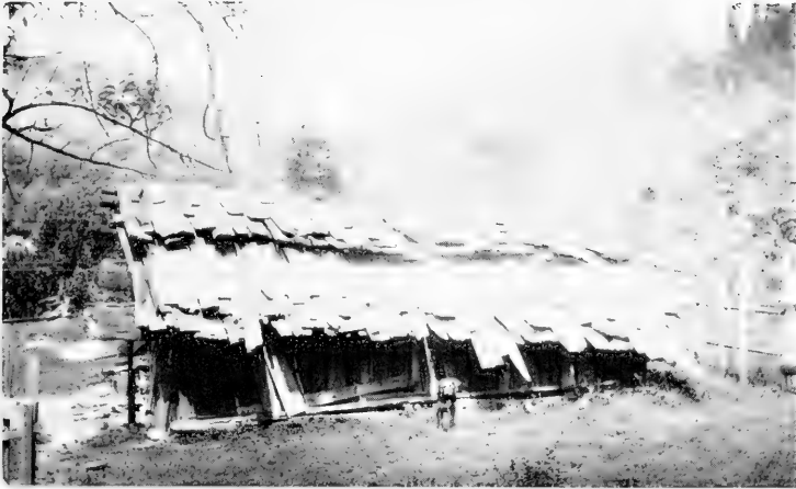
Karok plank house, showing double pitch and ragged shingling of roof. Northern California
