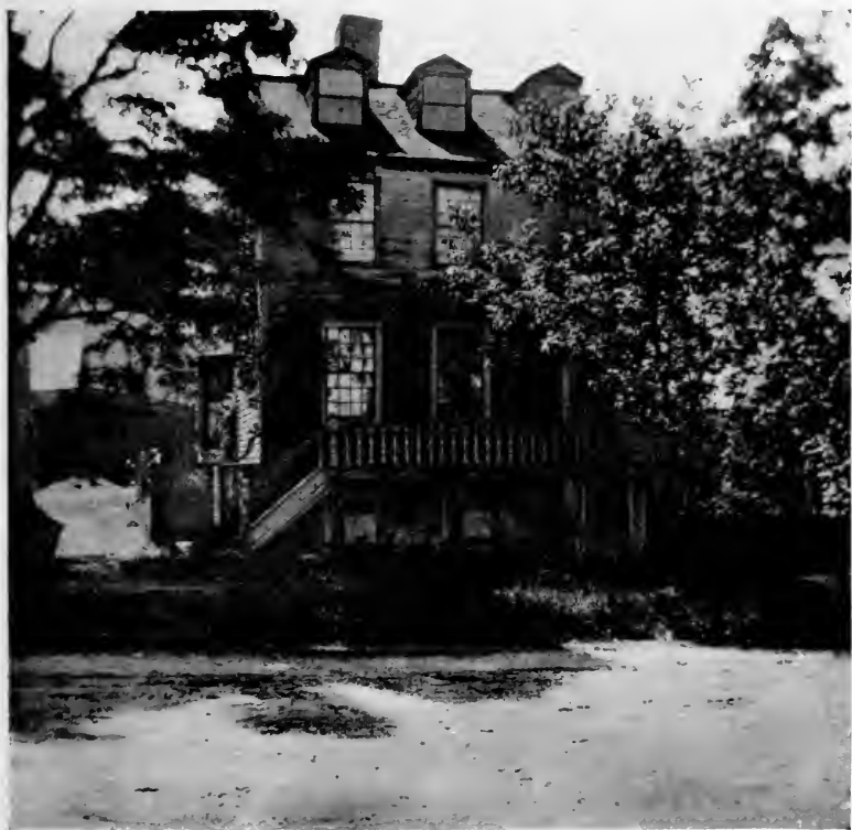
THE OLD GOVERNOR'S HOUSE, SHELBURNE.
