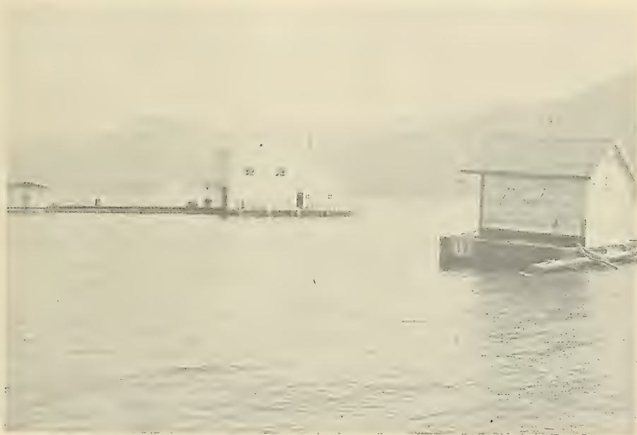
Figure 9. Installation at Lake Pend Oreille for deep-water tests, showing extension dock used to lower power and control cables into water. Small float in foreground holds transformers for boosting shore power to barge.
