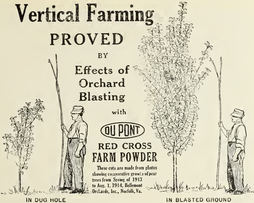
IN DUG HOLE
