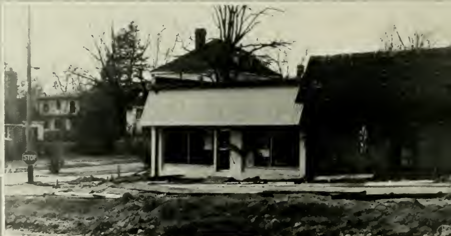
Top and bottom: Workmen level off ground for the new parking lot at the corner of Church and Mash Street
