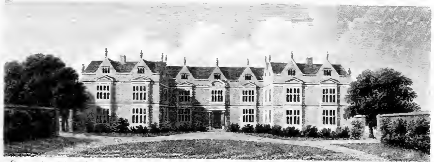
End added by Brown. Original South front. End added by Brown.
