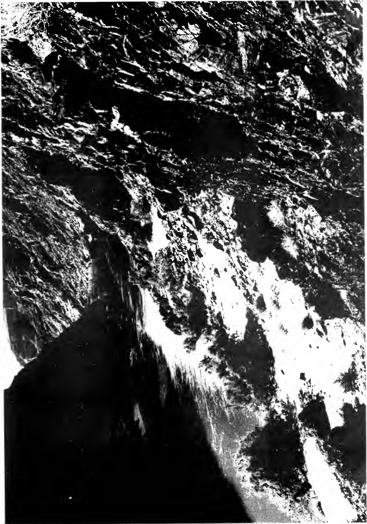
Figure 11. Bridge Canyon dam site, river mile 238, left bank.
