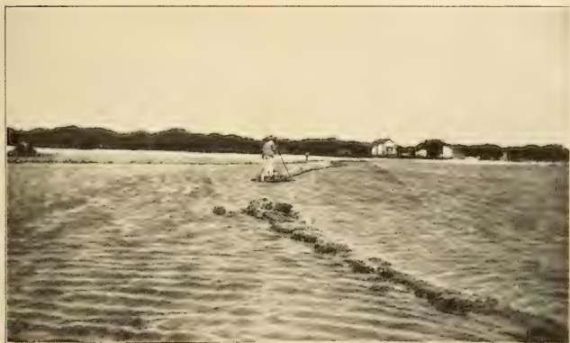
FIG. 10. NORTH WALL OF PAKULE, LOOKING WEST.
