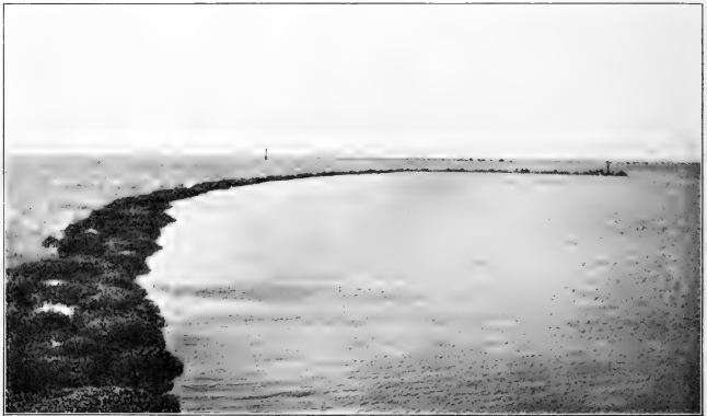
FIG. 9. OUTER WALL OF PAKULE, LOOKING SOUTH.
