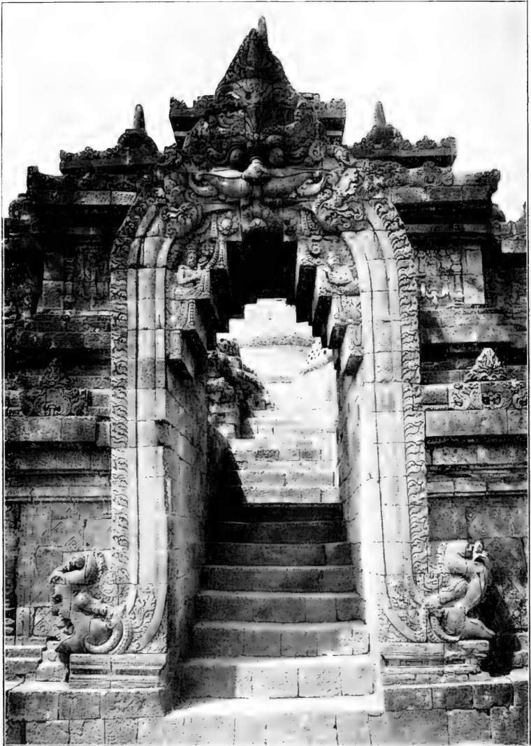
126. ONE OF THE STAIRWAYS.
