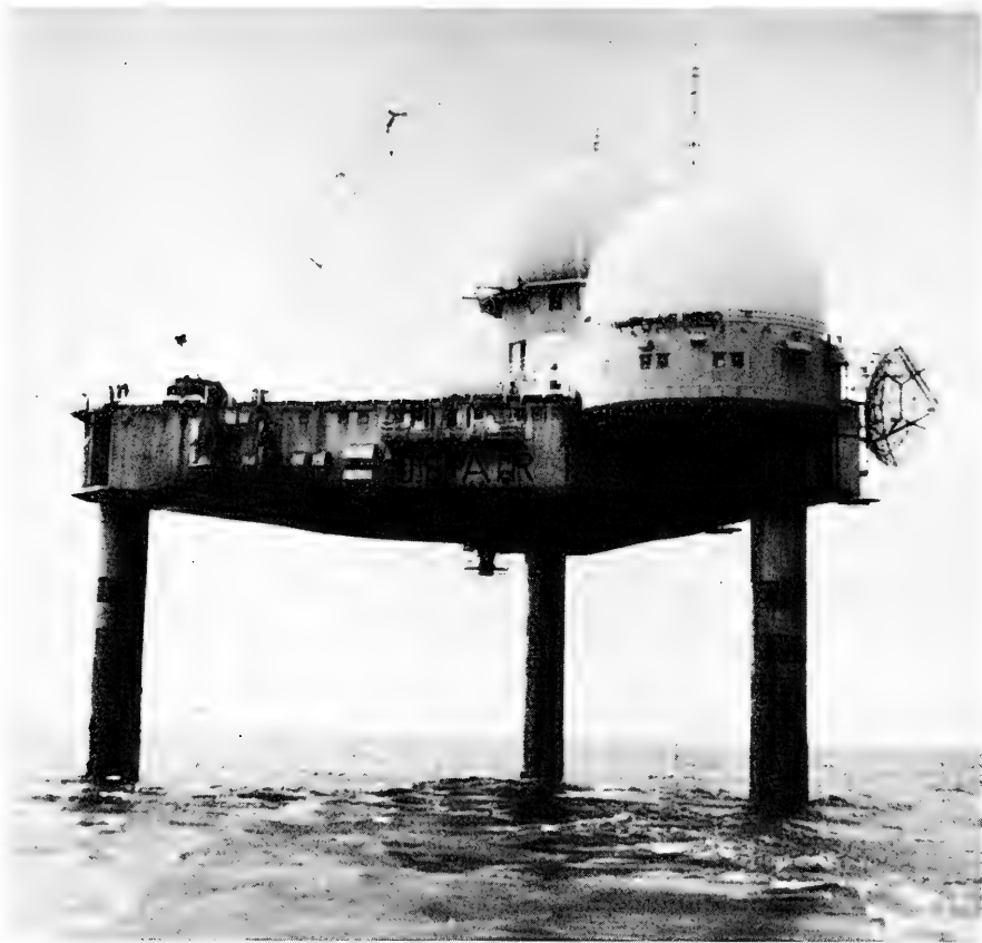
FRONTISPIECE—TEXAS TOWER NO. 4 OFF NEW YORK (COLLAPSED 15 JANUARY 1961)
