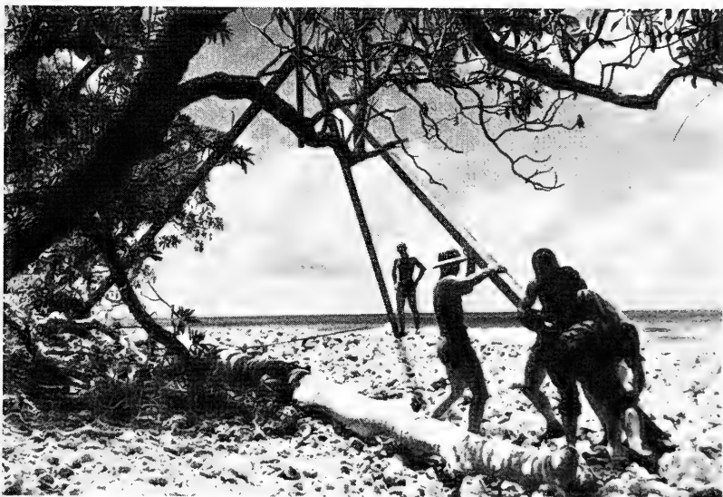
Construction of hydrographic signal on a remote island in the Pacific Ocean.
