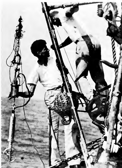
Dr. Watson with the Watson current meter. A. C. Woodcock at right.
