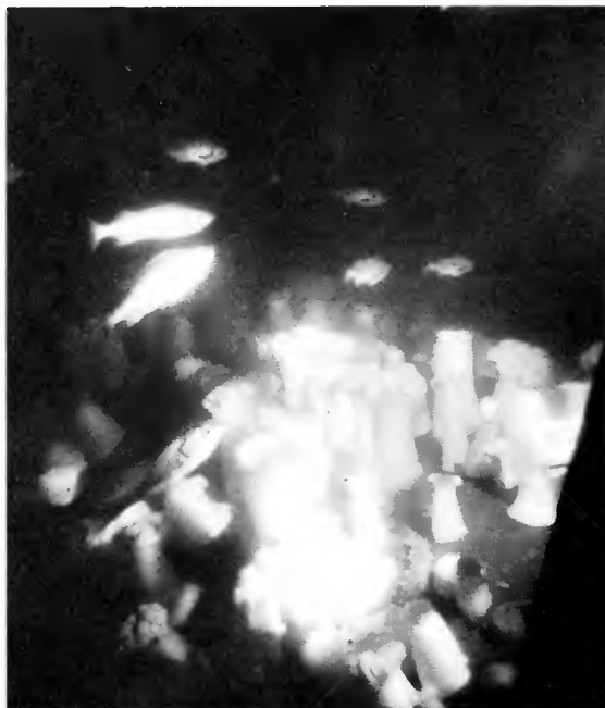
Section of outfall pipe near discharge outlet in Santa Monica Bay, California. Area is nearly five miles from shore. The white (colonial) animals on top of pipe are Metridium senile. Fish are various Sebastes. (Photo courtesy William Bascom, Southern California Coastal Water Research Project)
