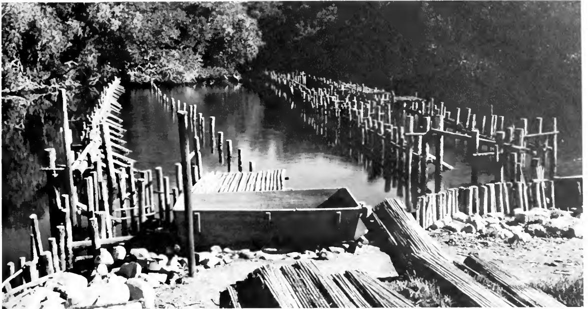
A weir (called a tapo) on the Estero El Mezcal, south Sinaloa. This weir, which belongs to an inshore fishing cooperative, is not in production. Its fencing has been rolled up and placed on the shore (foreground) so it will not rot. (Photo by author)
