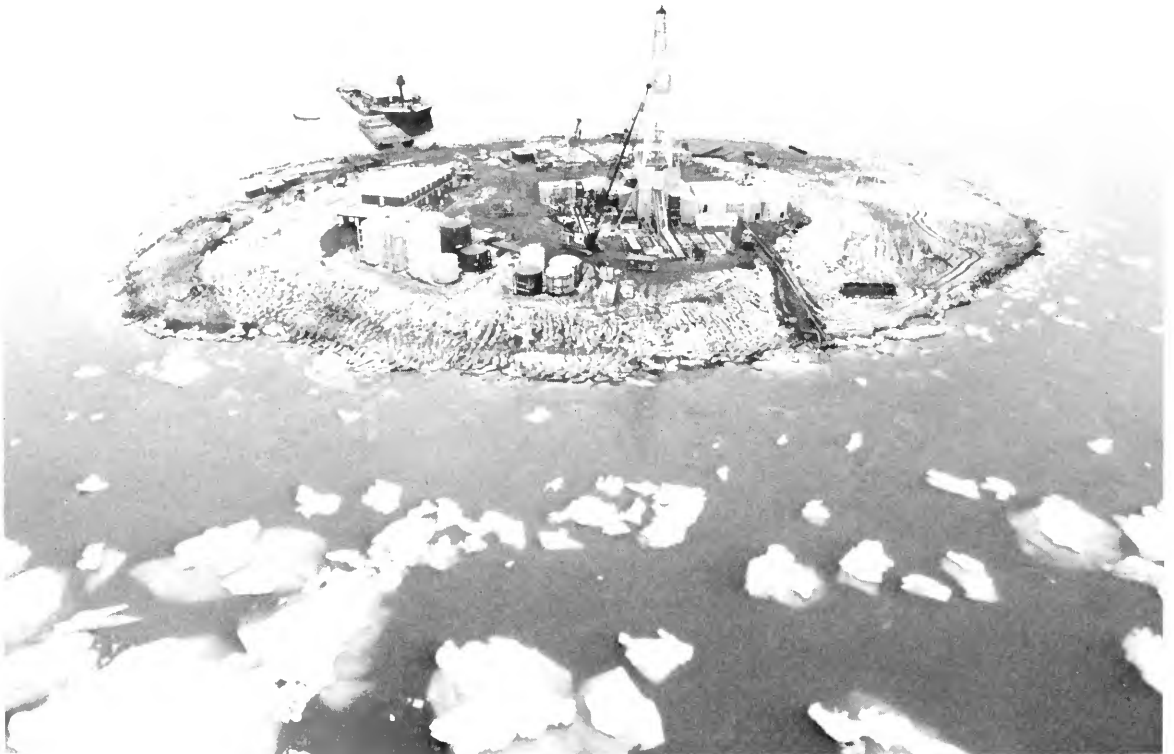
Issungnak Island in the Canadian section of the Beaufort Sea in September. This is a "sacrificial beach" island; the outer rim breaks storm waves in summer and causes ice sheets to break up and form a protective rubble field around the island. Sandbags and filter cloth reduce erosion. The island is made of 4.9 million cubic meters of sand, dredged from the seabed and delivered to the site through a floating pipeline. It is 26 kilometers offshore in water 19 meters deep. From November through June, there is no open water around the island. In the winter, the sun does not appear on the horizon. (Photo courtesy of Esso Resources Canada, Ltd.)
