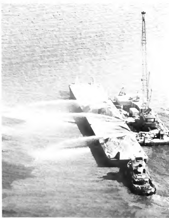
Clam shells on a barge are sprayed by high-pressure hoses into water off the coast of Louisiana. Funded with a federal grant under the Coastal Energy Impact Program, this project provided material on which larval oysters could attach themselves, thus rehabilitating or relocating oyster reefs which were damaged by petroleum industry activities. (Photo courtesy of Louisiana Department of Natural Resources)
