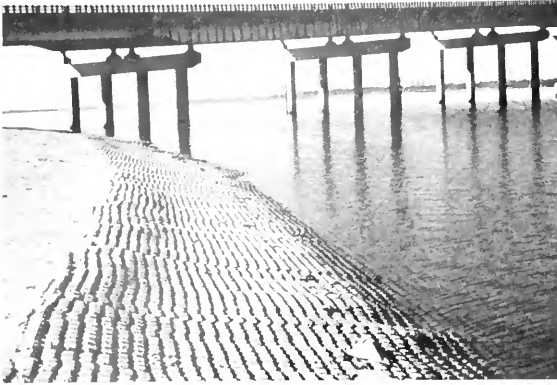
Riprap prevents further erosion at a small park in Calcasieu Parish, Louisiana. Wake from ship traffic in a nearby ship channel had eroded the park's beach. Because the ships were travelling to and from petrochemical plants that were built because of oil rigs offshore, the state of Louisiana applied for and received a federal grant under the Coastal Energy Impact Program. The money was used to restore the beach with sandfill and riprap and to purchase picnic tables. The park is popular with the employees of the nearby oil refineries. (Photo courtesy of Louisiana Department of Natural Resources)
