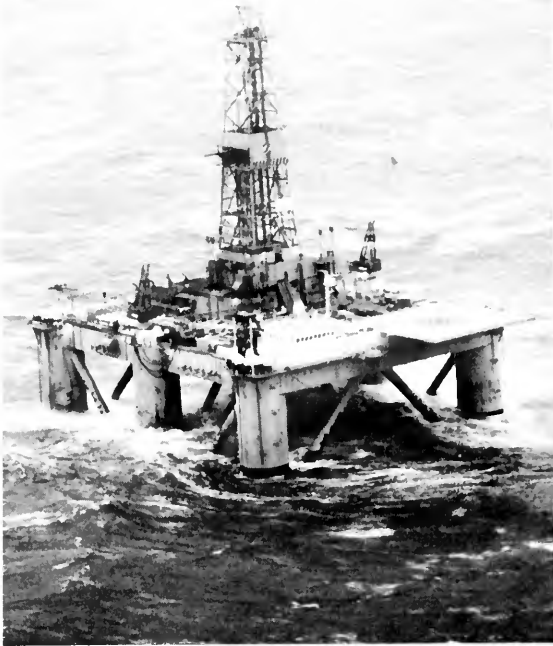
As oil exploration pushes farther into the stormy waters of the North Atlantic, greater risk to life and property must be anticipated. Above, a drilling rig in rough weather. (Photo courtesy of Tenneco)
