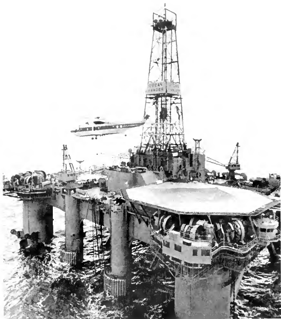
Deeper drilling implies greater danger. The Ocean Ranger, a 37-story-tall behemoth, was considered unsinkable. When it went under in 100-mile-per-hour winds off the coast of Newfoundland, 84 people died. (Photo courtesy of UPI/Bettmann Archive)
