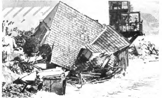
A West Coast house destroyed by storms (L.A. Times photo)
