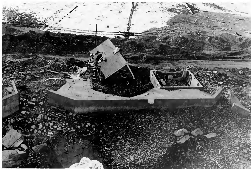
A Scituate home after the storm had passed. (Photo courtesy of the Federal Emergency Management Agency)
