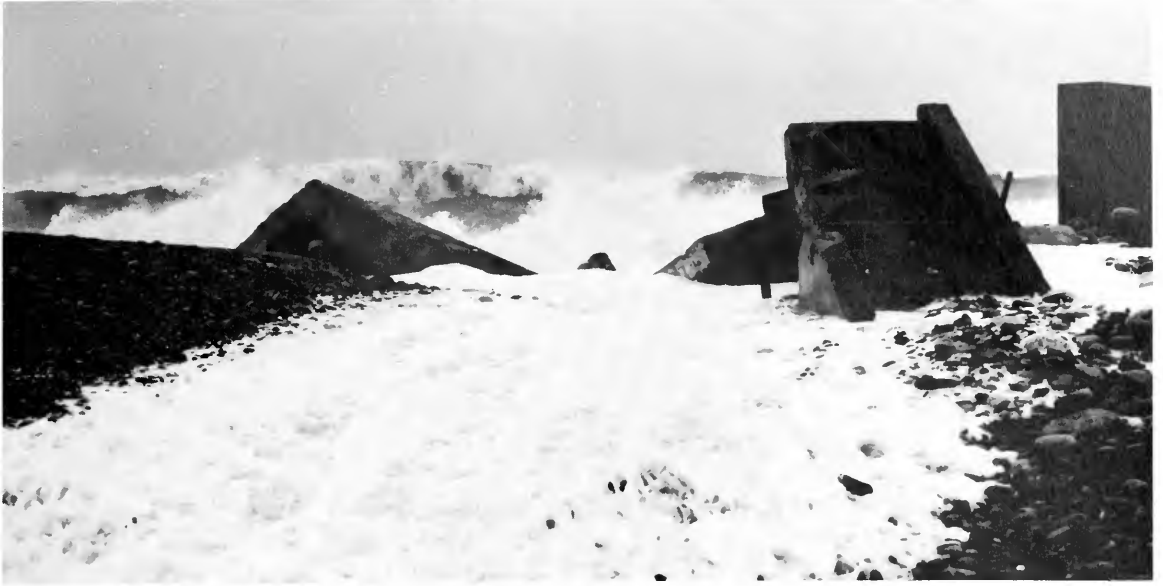
In 1984, waves crashed over these remains of a house destroyed by another storm in 1978. The land was purchased by the federal government under a pilot program of buying storm-damaged property covered by federal flood insurance rather than paying to have it rebuilt. The land is now administered by the state and the local community as public open space. Had this home been rebuilt, it might have been destroyed again last year, and the government again would have been responsible for the cost. (Photo by Jeff Benoit)
