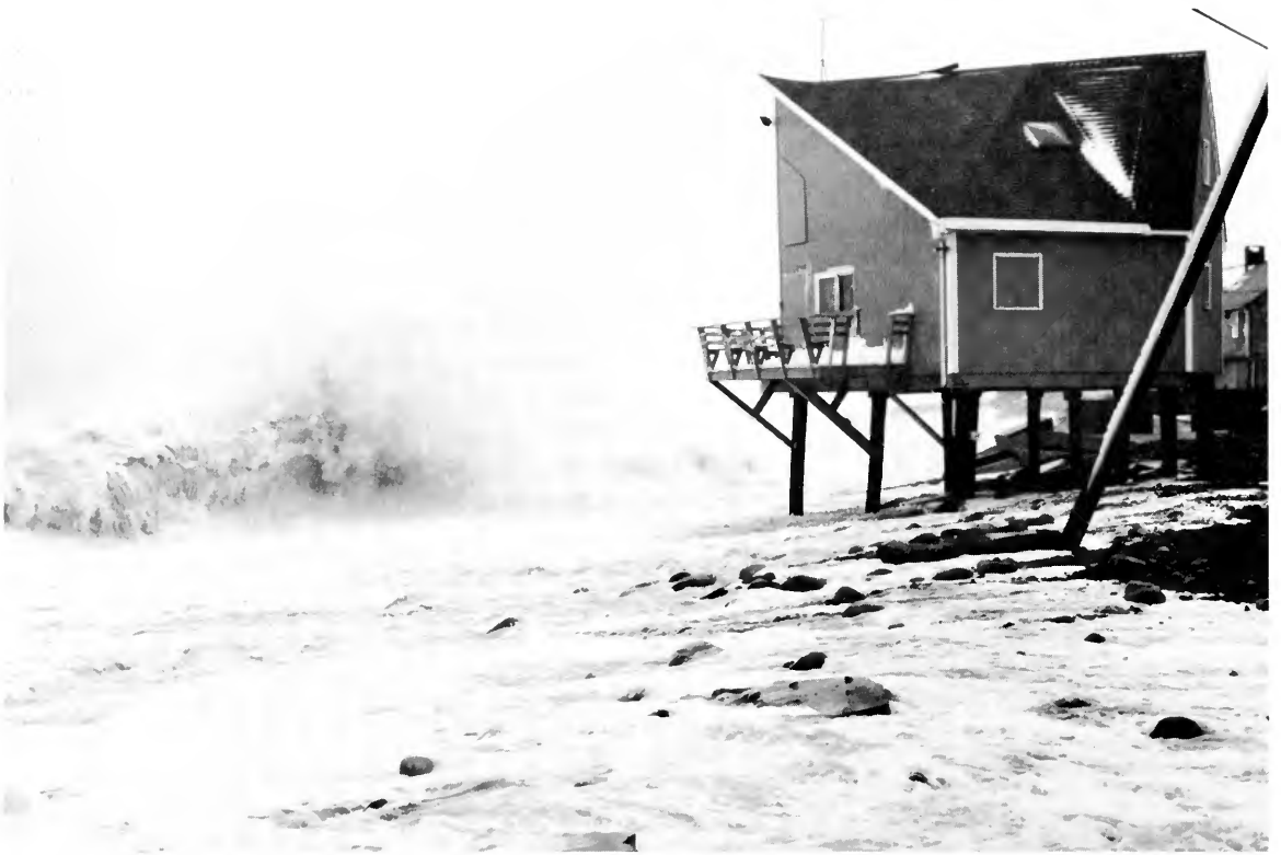
This house was severely damaged by a storm in 1978. When rebuilt, it was raised on pilings so that storm waves pass under instead of through it. The extra care proved its worth in the 1984 storm shown here. As sea level rises, however, the coastal barrier on which the house is built will retreat, and the house will seem to move out to sea. Such storm-proof structures eventually impinge on both the aesthetics and recreational utility of the beach. (Photo by Jeff Benoit)
