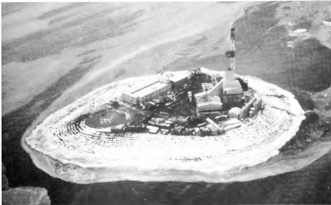
The largest man-made gravel island ever built in U.S. waters. Called Mukluk, it is located 65 miles northwest of Prudhoe Bay in the Beaufort Sea. (Photo courtesy American Petroleum Institute)
