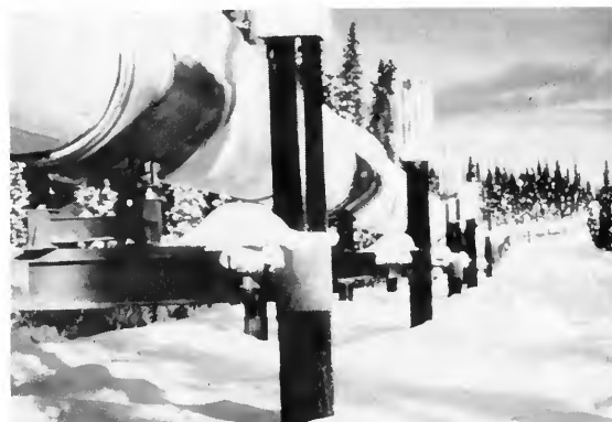
The trans-Alaska pipeline in winter. (Photo courtesy American Petroleum Institute)
