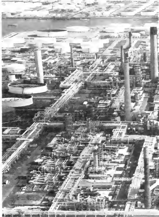
The petroleum storage tanks at Rotterdam are linked by pipeline to 14 refineries in Belgium, the Netherlands, and West Germany. (Photo by B. Hofmeester)
