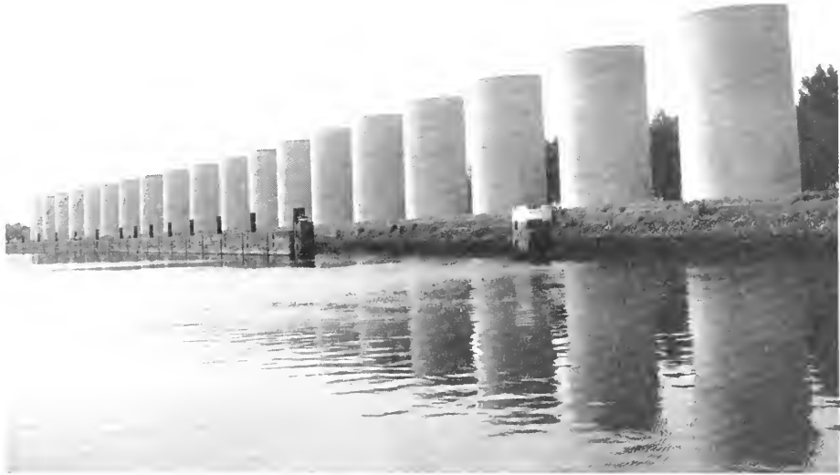
The Calandbrug Wind Wall cuts the force of heavy winds, permitting a higher traffic flow through the port. (Photo by the author)
