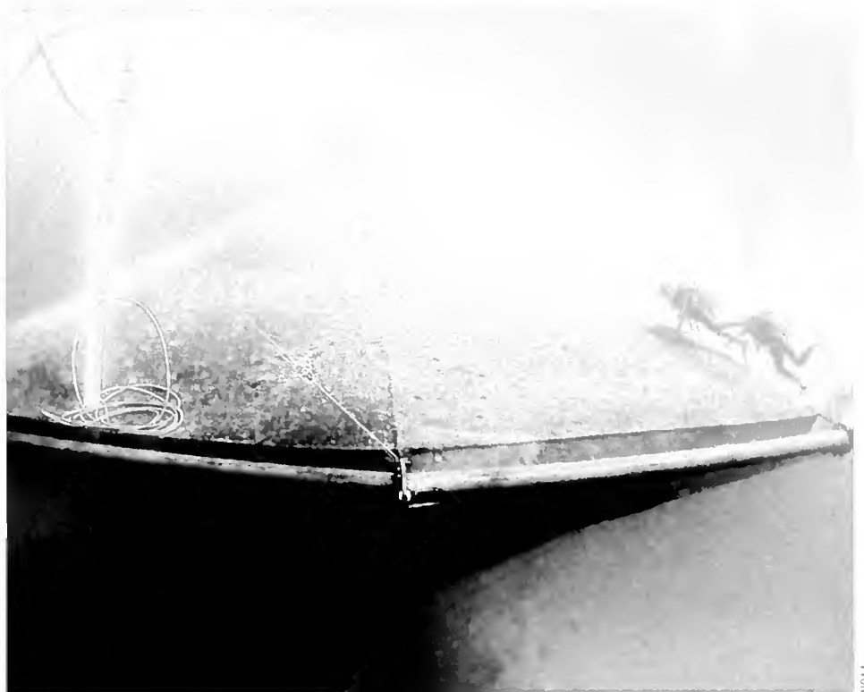
▲ Divers clean the outside of SeaStation 3000, an open-ocean aquaculture project operated by the University of Hawaii. The 15-by-24-meter (50-by-80-foot) cone-shaped steel-and-mesh cage lies two miles from Honolulu and 12 meters (40 feet) below the surface, out of the way of ships.
