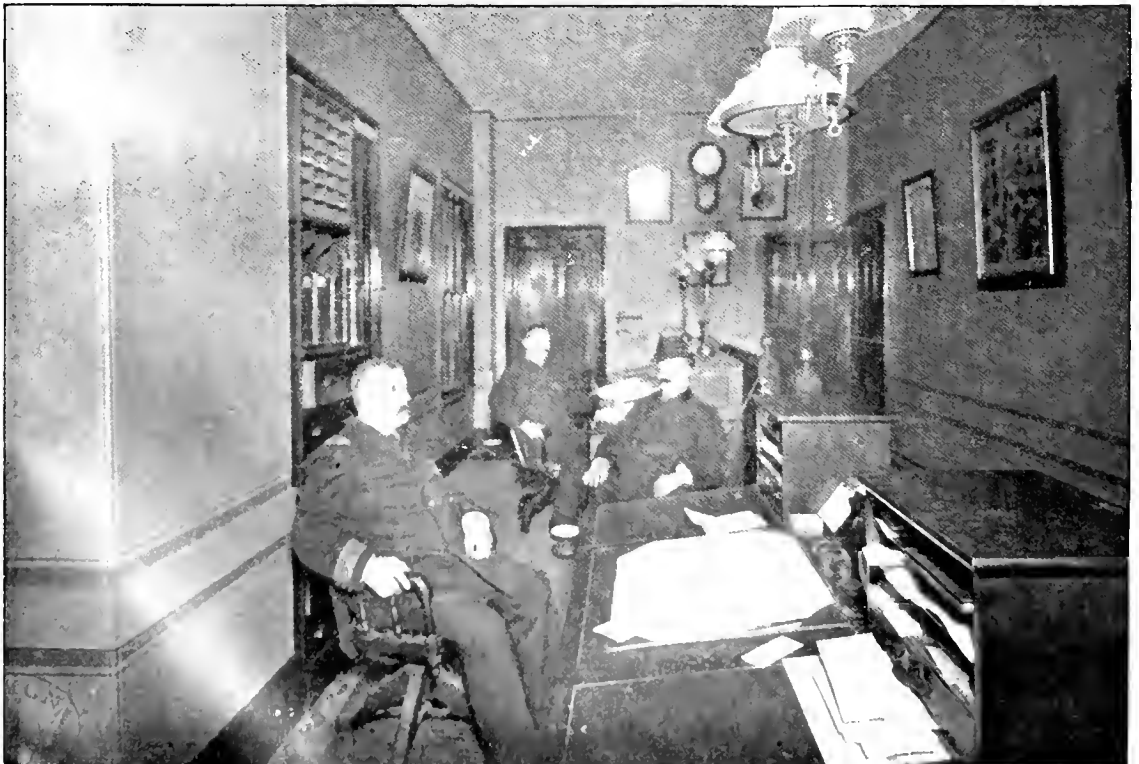
INTERIOR OF DIVISION THREE.
