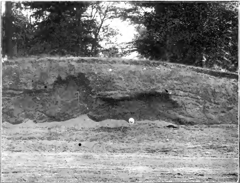
FIG. 6. A portion of the cross section on the south side of Sixteenth Avenue.
