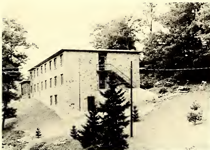
McAlister under construction in 1958.
