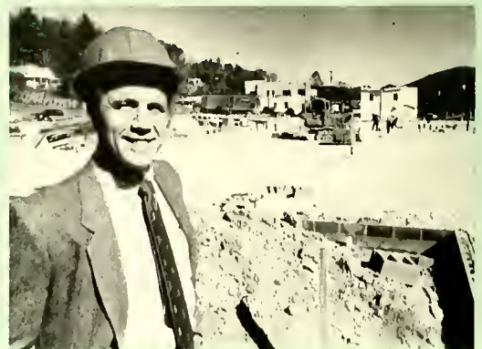
Dr. Crain views the foundation for the new structure.
