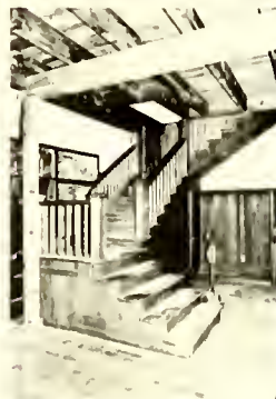
The historical landmark on campus. "Hemlock Hall," formerly the residence of the hall sisters of Wilmington (Cheeononda), underwent a transformation this year. At left, a view of the structure before restoration took place. LMC maintenance personnel conducted the remodeling and refurbishing of the 80 year old structure. (Above right, next page) The new deck and the refurbished greatroom and sunporch provide a renovation that makes the original building unrecognizable. Open house for the 1988 graduates and parents was held in May as the official opening of "Hemlock Hall"
