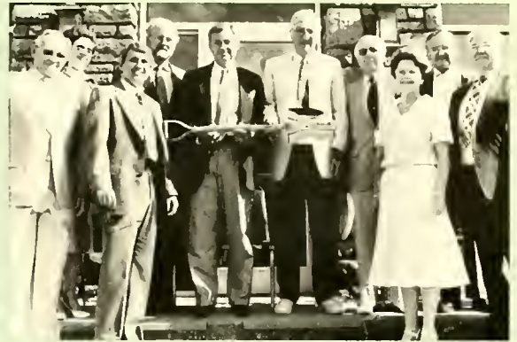
Trustees Faw, Huffine, Massie, Clement, Hathaway, Lovell, Walrath, Melton, McCarl, Hale, take part in groundbreaking.
