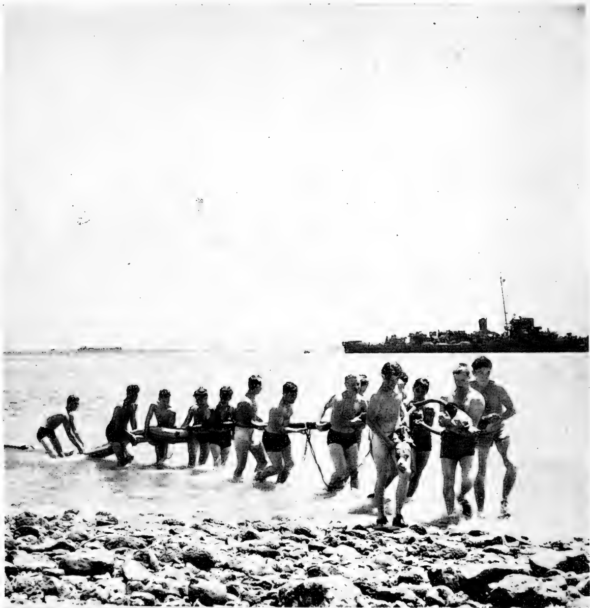
OPERATION KILOWATT HOUR. At Kwajalein Island, during an important period in the preparatory phase of the atomic tests, electric power on the island, normally supplied by two 250-kilowatt generators, suddenly failed, with no possibility of repair until special parts had been obtained from the United States. To bridge the gap a destroyer equipped with special generator facilities was dispatched to Kwajalein, to serve as the Kwajalein supply for as long as necessary. Shown above, amphibious members of the 2,750 Air Corps personnel stationed in the Marshalls bring ashore from a power boat (not shown) the end of an electrical cable extending under water to the destroyer in the background.
