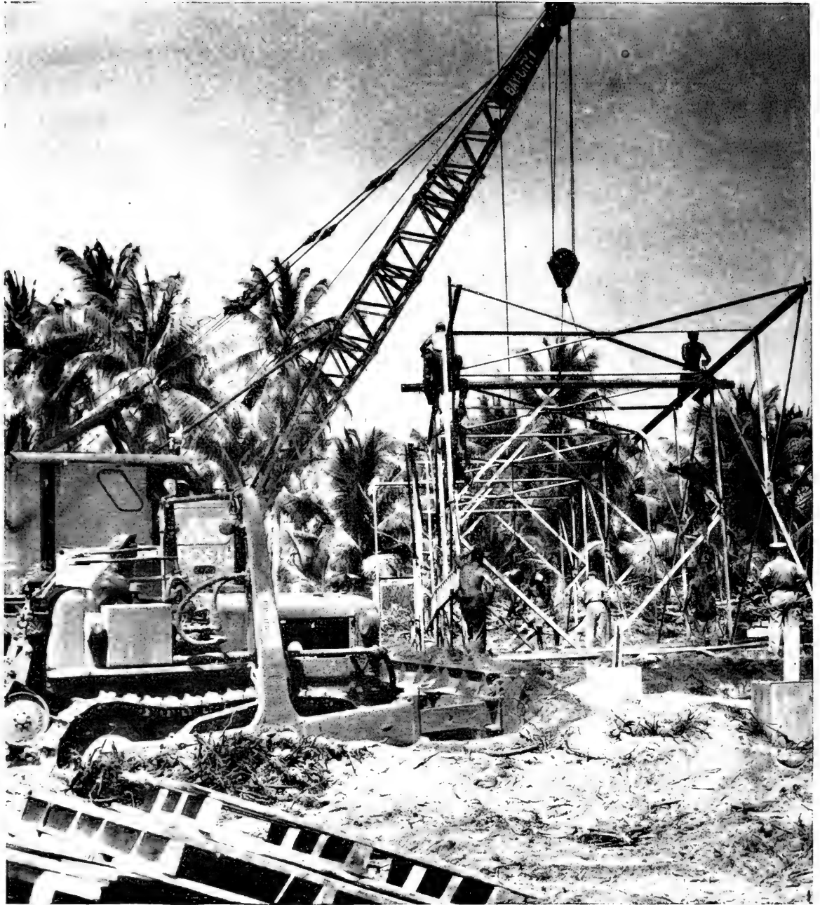
INSTRUMENT GRANDSTANDS GO UP. Instruments, the eyes of the Operation, were installed on top of steel towers erected on various islands surrounding the Bikini lagoon. Television cameras mounted in these lofty grandstand seats were focussed on the target array and, when the tests occurred, permitted scientists miles from Bikini to witness what was going on at the test site. Still and motion picture cameras were also berthed on top of towers to make a permanent photographic record of what occurred. Towers were assembled on the ground and hoisted into place.
