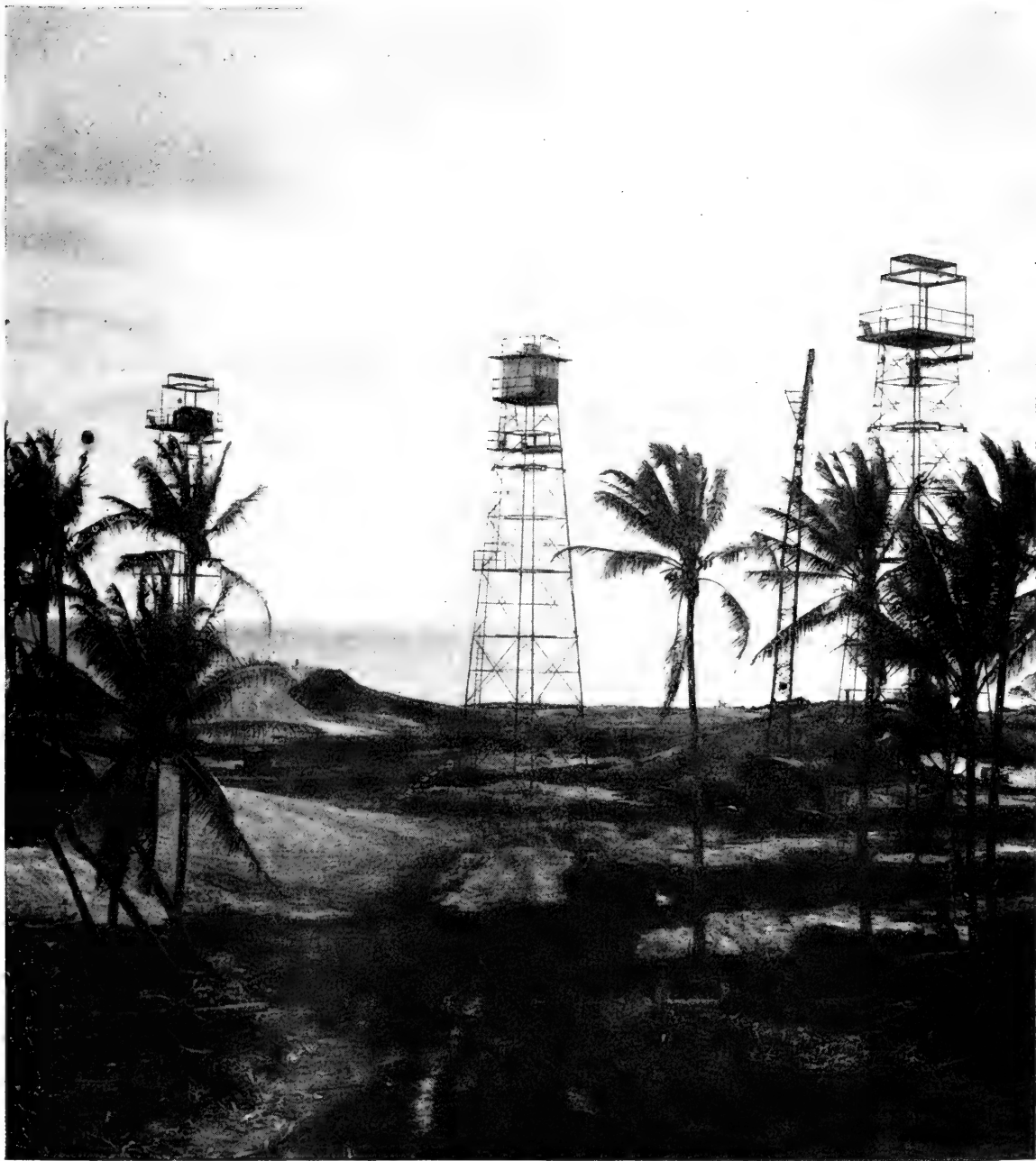
TOWER GROUP, ENYU ISLAND. A further view of the types of tower installations made to house delicate apparatus used to record the characteristics of the blasts. Many of the photographs in this volume and many of the best newsreel views of the explosions were taken from towers such as these. Cameras were installed inside lead-walled vaults, the doors of which were arranged to close automatically after the filming had been accomplished, thus protecting film from the harmful effects of gamma radiation. Each tower amounted to an extensively equipped observation station..
